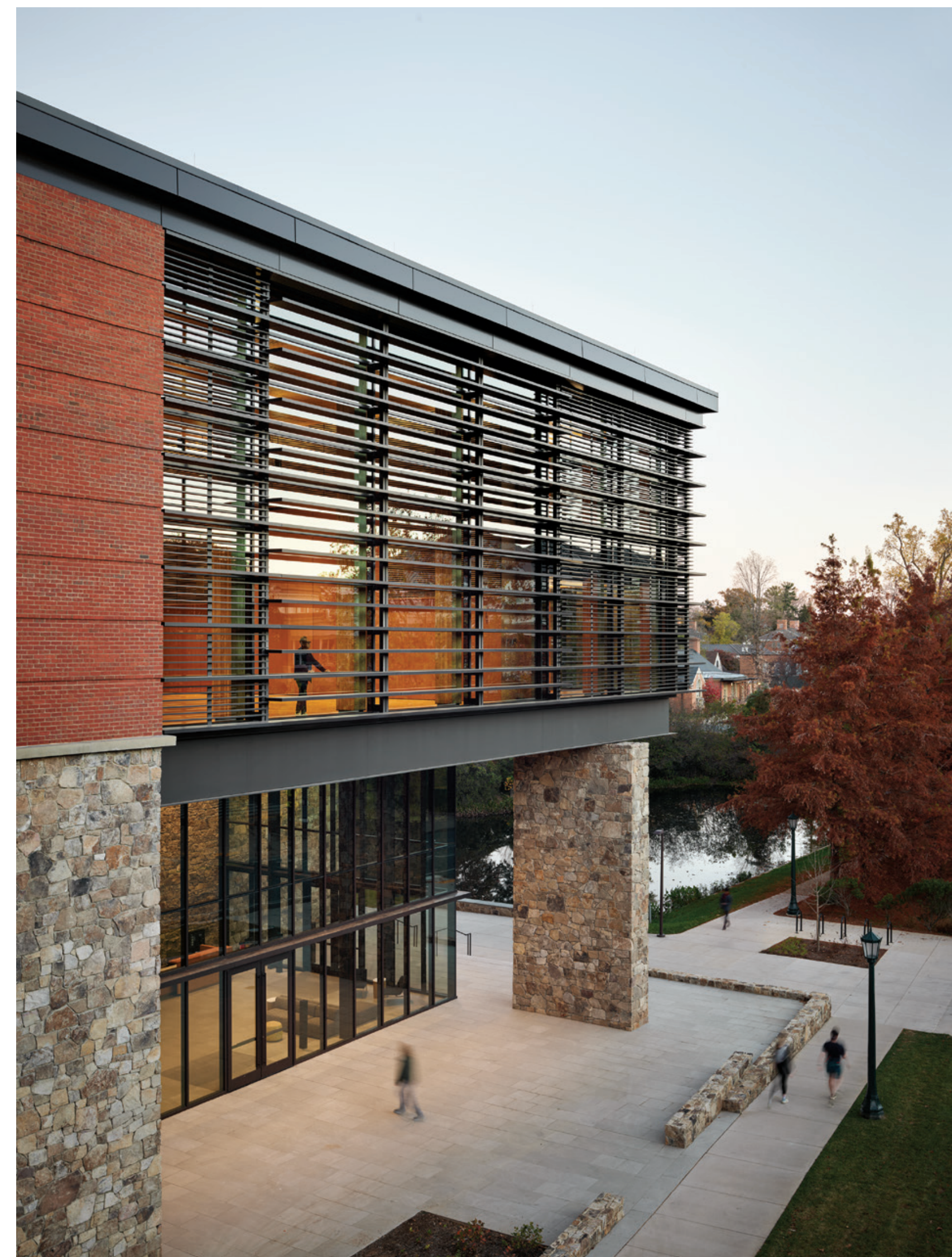
Parts of the facade (above) and ground-floor lobby (opposite) include biophilic materials such as wood and fieldstone.
