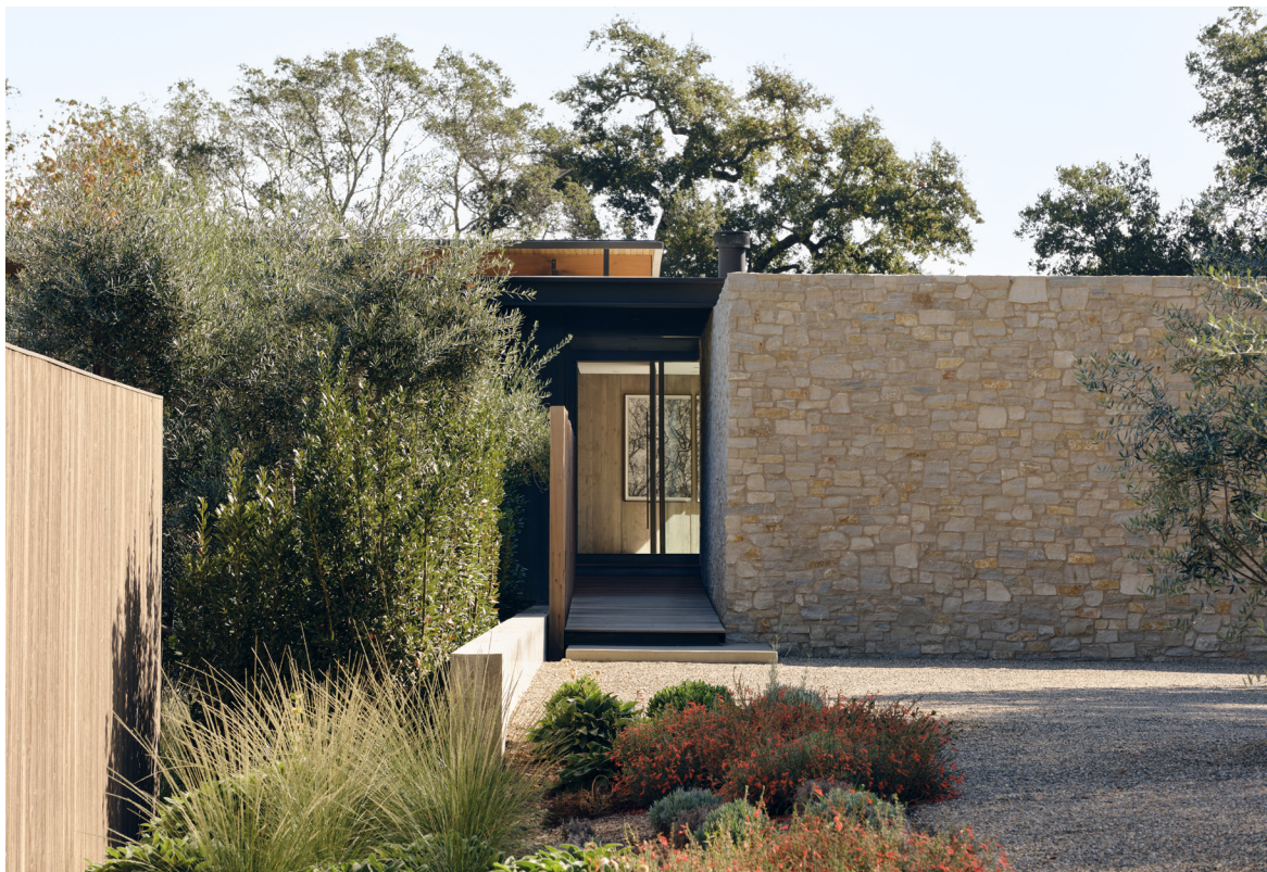
ABOVE: The front door is accessed by a boardwalk tucked behind the carport, which was clad in local fieldstone. The architects chose hardy, low-maintenance building materials that would acquire a patina over time. ADAM ROUSE PHOTOGRAPHY
